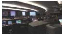
2 Operational Control Centers
