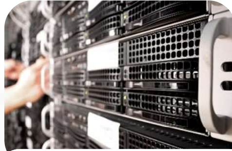
Construction of System/Network
